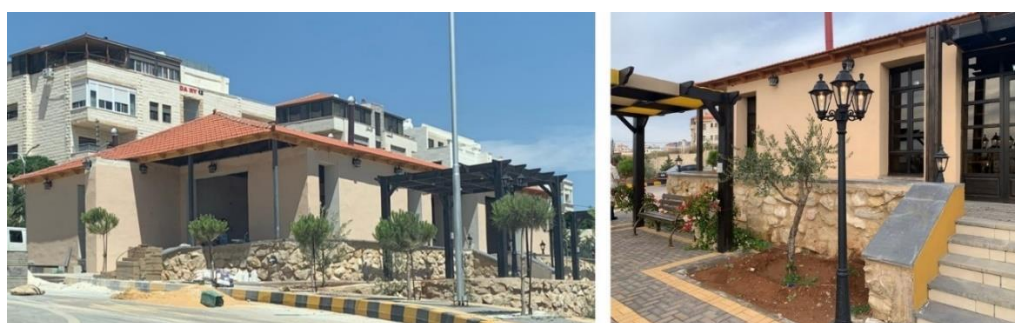
Figure 10. The completed rammed earth building
