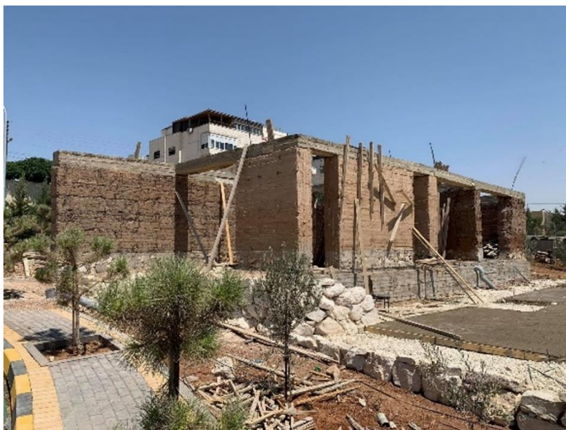
Figure 8. Rammed earth walls after removing the formwork.
