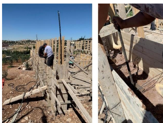
Figure 7. The construction of rammed earth walls.
