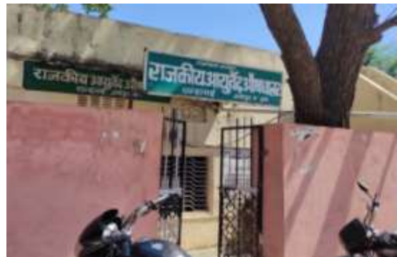
Government Ayurveda Health Centre, Chandlai
