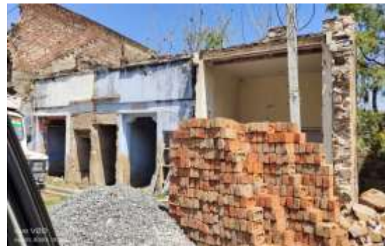
Old Residences converting into Shops, Chandlai
