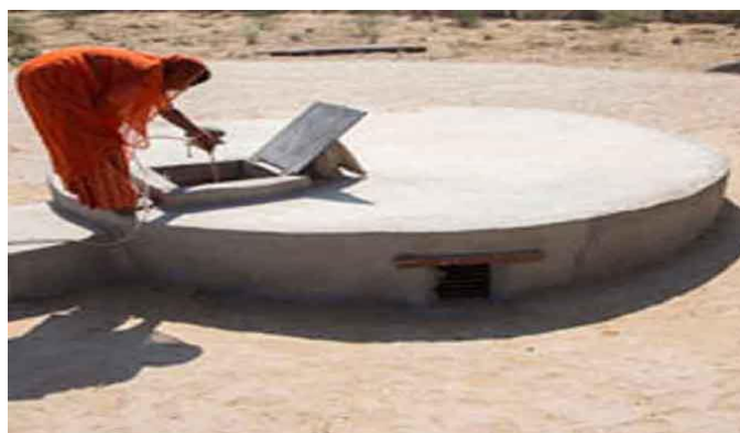
Fig. 9: Picture showing underground tanka
