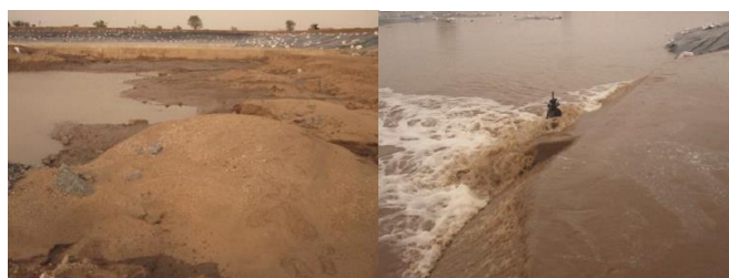
Fig. 15: Heavy siltation due to high-run-off
