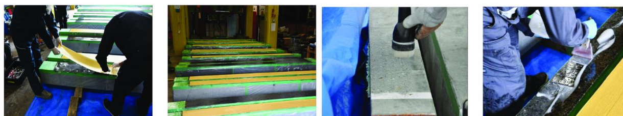
Figure 20: Surface treatment, epoxy resin application, AFRP sheet bonding, completion & curing
