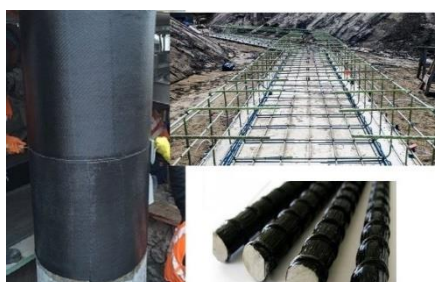
Figure 19: CFRP applications in the structure
